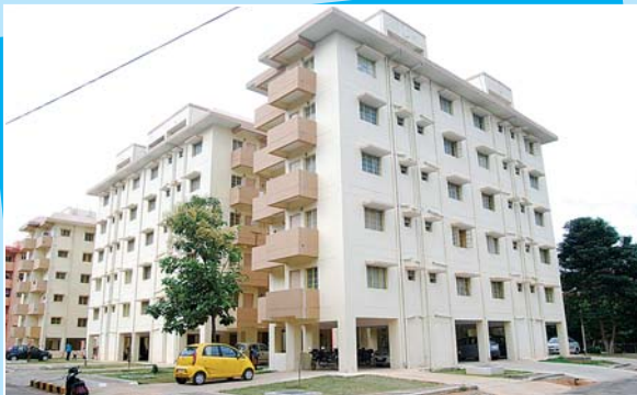
Building Works at HAL, Bangalore
