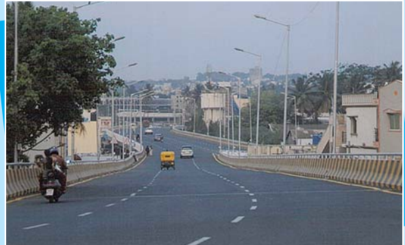
GATF Flyover, Bangalore
