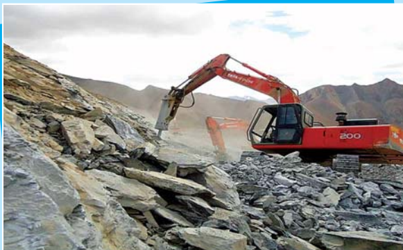
Hard Rock Cutting by Breaker at Leh
