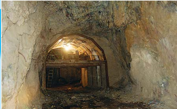
Tunnel Work at Hathiri Power House, Uttarakhand
