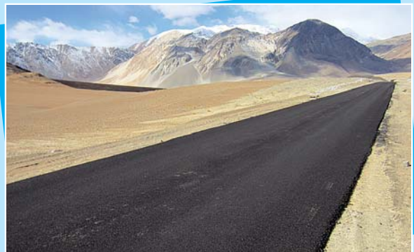
Road Work at Leh
